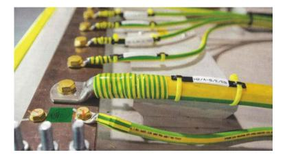
All equipment, equipment grounding lugs, and metal cabinetry should be bonded to a common ground point. Ground the equipment cases but not the internal supply wires. Notice the universal color code recognized throughout all North American jurisdictions: **Green** can only be used for equipment grounding and never for anything else. This requirement is simply to insure any future installer will always be confident that line cannot be anything else except a path to earth.
