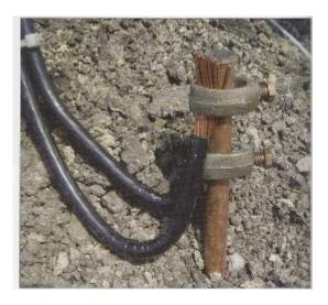
**Equipment grounding conductor size** should be at least 14 Ga. NEC Code wants 8 Ga for lightning protection and you'll find 14 Ga or 12 Ga equipment grounding conductor size in all installations made during the past ~5 years.
