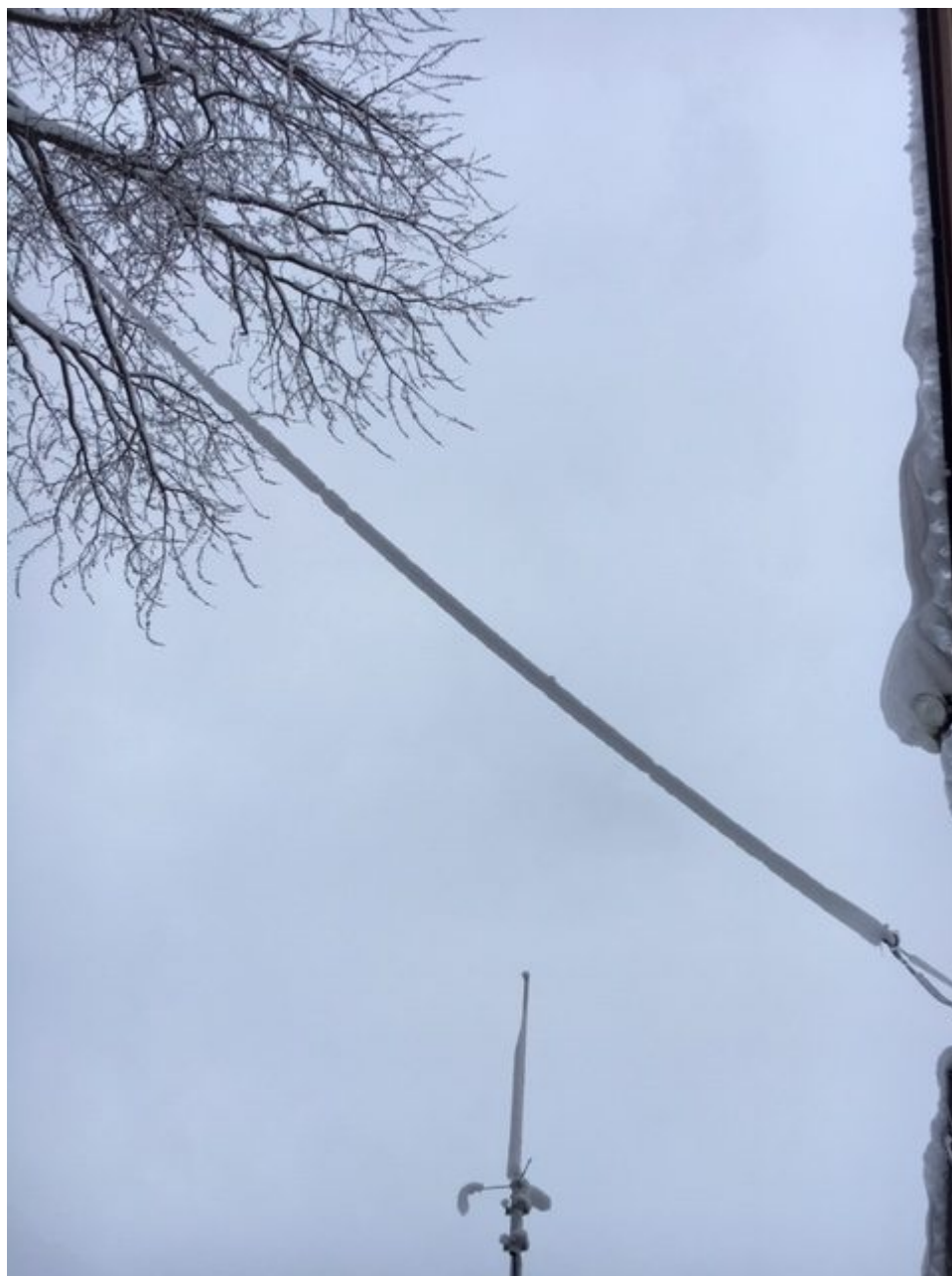
A wire antenna KD9KMV has grown significantly in diameter with ice
